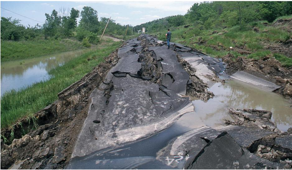
Figure 5—A section of McDowell Creek Road just south of Manhattan, damaged by a landslide after heavy rains in the spring of 1995. The roadway was displaced about 20 feet vertically and 40 feet horizontally.
