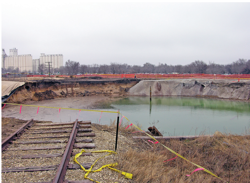
Figure 1. Filling the 1974 Cargill sinkhole caused by salt removal in Hutchinson in Reno County. Around humanmade infrastructure, sinkholes are not just hazardous; they can cause immense economic damage and block transport channels.
