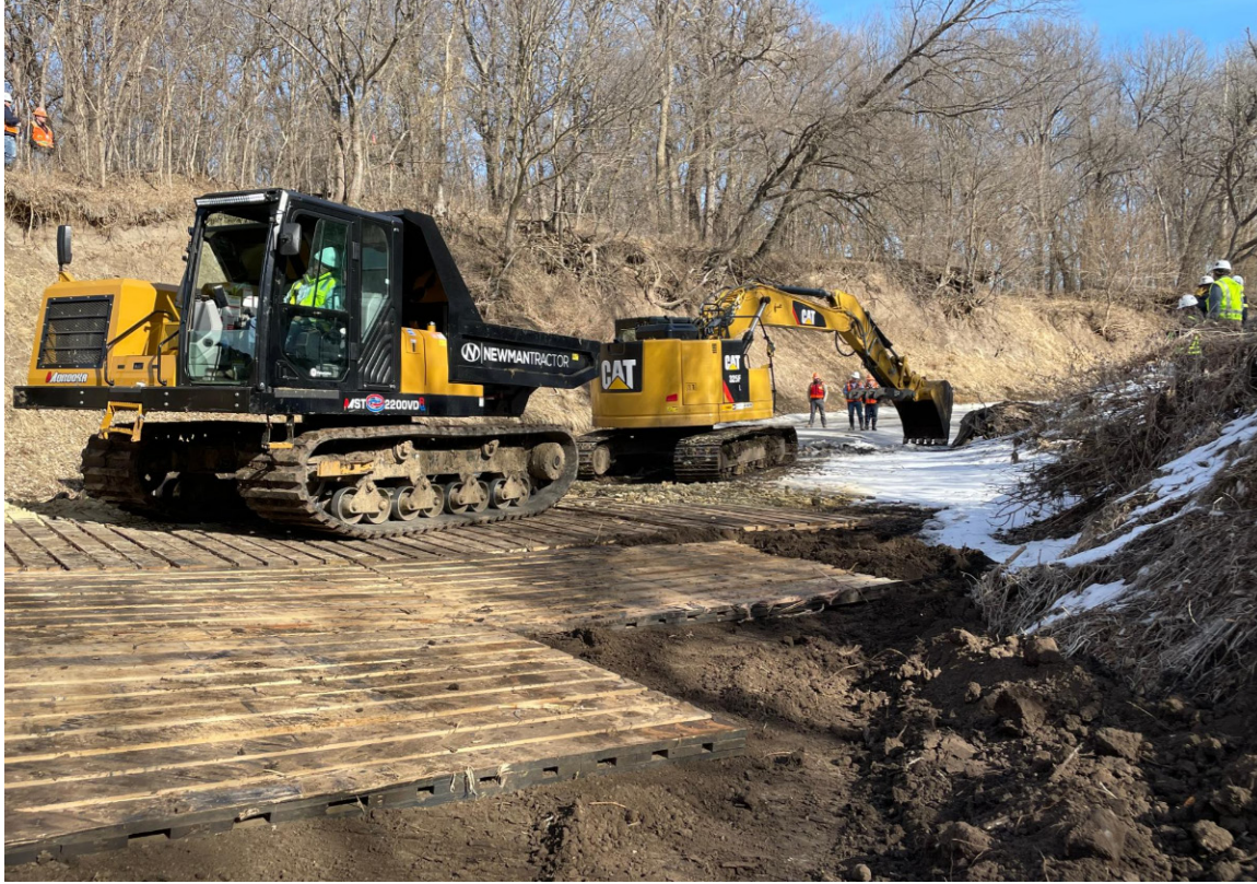
Figure 5: Construction workers remove and treat contaminated soil at Mill Creek. Photo: Environmental Protection Agency.
