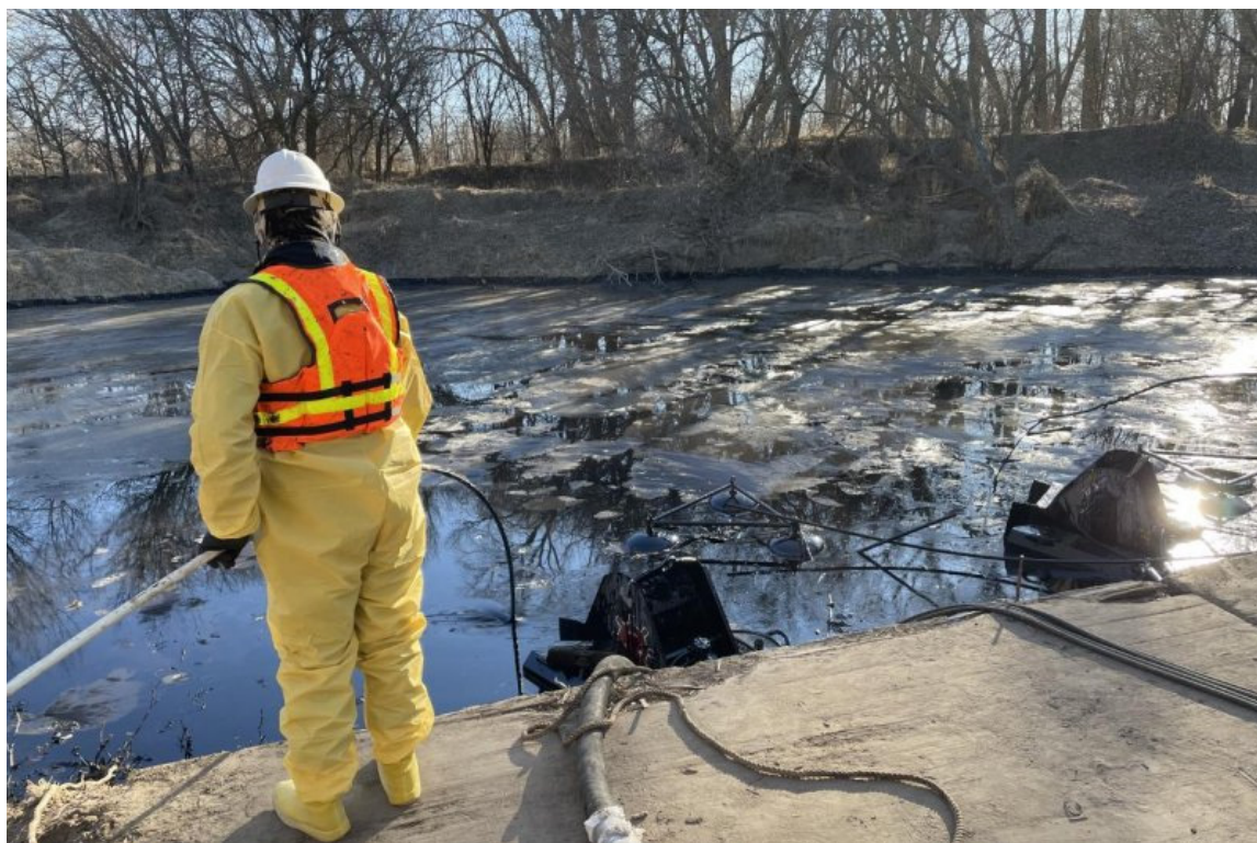
Figure 2. A construction worker uses skimmers to pump oil out of Mill Creek. Photo: Environmental Protection Agency.
