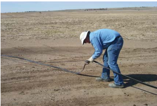
Figure 42. Installing cable protector across road.
