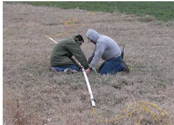
Figure 106. Engineering technicians Andrew Newell and David Thiel prepare the Ethernet cable shield for insertion into a culvert under the east/west county road.
