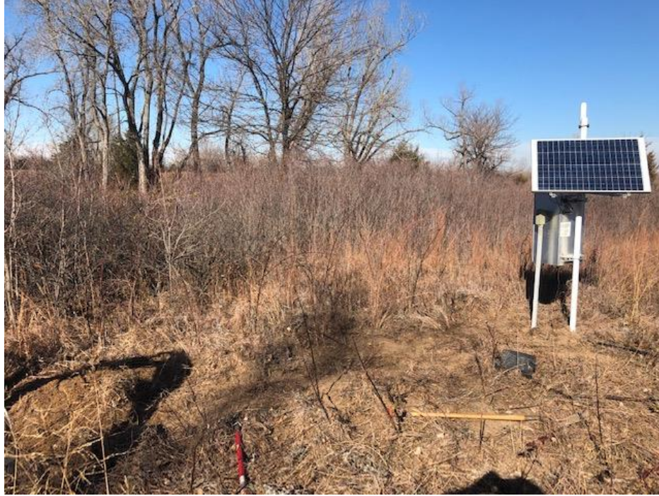
Figure A-11. RN03 is located in Reno County northeast of Hutchison in Sand Hills State Park. It is installed about 2.5 mi from Kansas Highway 61.
