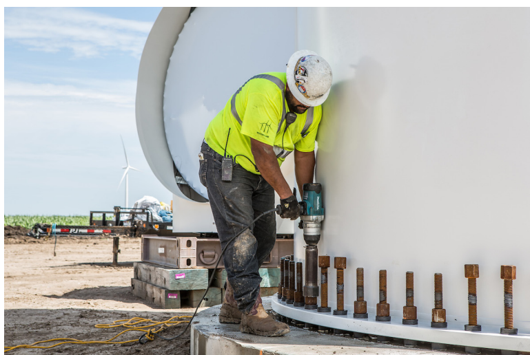
Figure 6. Invenergy worker securing the base of the turbine to the surface pad. (Photo by Tim Nauman.)
