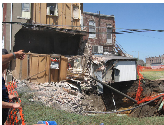
Figure 13. Sinkhole that opened in Galena in 2009. Damage to apartment building (top), and interior view of sinkhole (bottom). (Source: Kansas Department of Health and Environment Superfund Program.)
