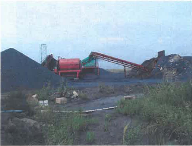
Coal crushing facility.
