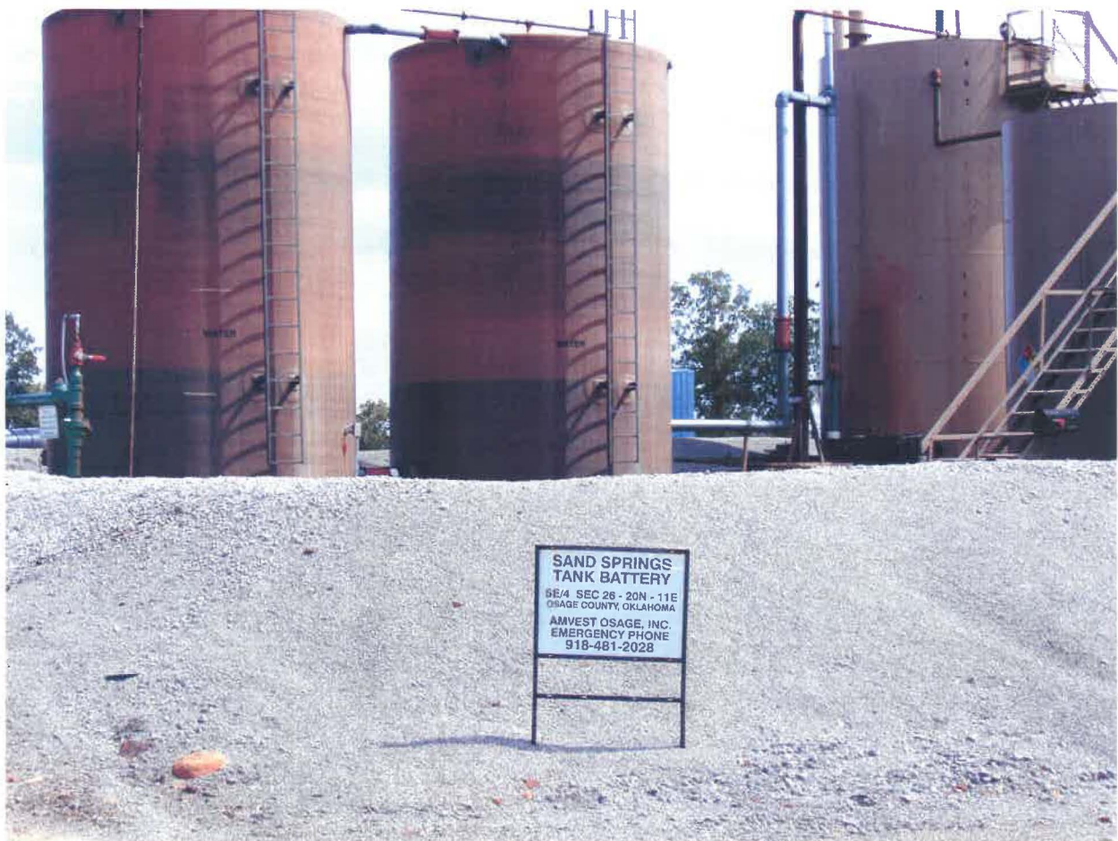
Amvest Osage, Inc. Sand Springs Tank Battery.
