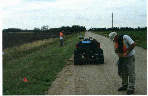
Fig A8. Winding cable along east road ditch of Victory Road south of U.S. 50.
