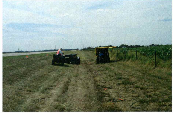
Figure 5. Receivers were "planted" at the base of the road ditch to insure highest possible quality coupling.
