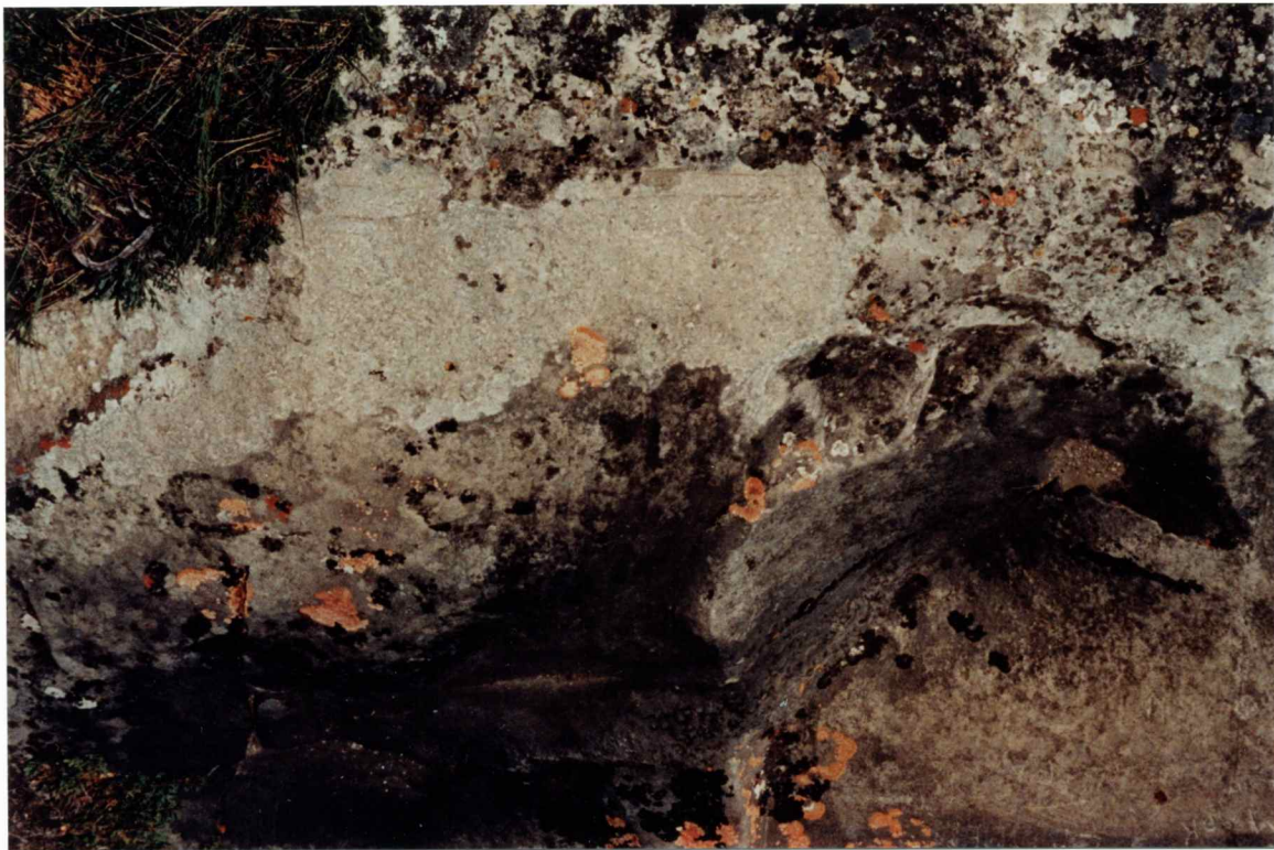
Figure 8. Most of the white (and red-orange) matter in the picture is lichen growth. Such growth is common at the St. Victor site.
