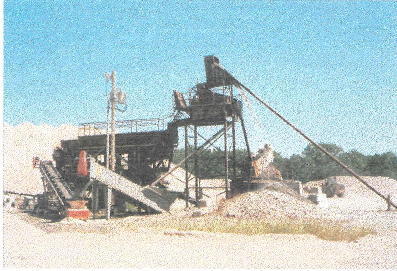
Figure 8. Sand hopper for a floodplain dredging operation. (Midwest Concrete Materials, Inc., Manhattan, KS)
