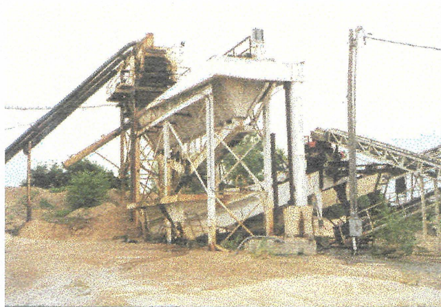
Figure 5. Sand hopper used to sort bulk sand. (Penny's Concrete, Lawrence, KS.)
