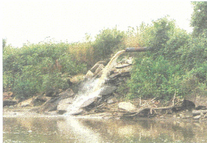
Figure 1. View of return pipe from the sand processing plant located at the Penny Concrete dredge site below Bowersock Dam
