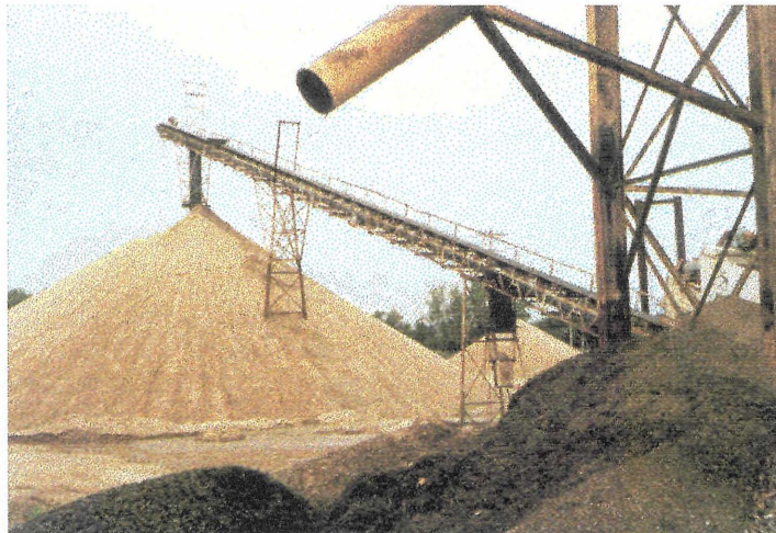
Figure 6. Conveyor belt from sand hopper to sand stockpile. (Penny's Concrete, Lawrence, KS.)
