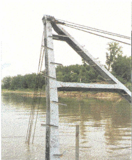
Figure 4. A-frame used to raise and lower the ladder auger. (Penny's Concrete, Lawrence, KS.)
