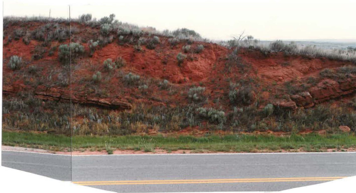
Figure 35: Dissolution collapse feature in Dog Creek Formation; north side of Rte. 160, approximately 14.5 miles west of Medicine Lodge, Barber County, Kansas; SC1/2, SW1/4, Sec. 6, T32S, R14W.
