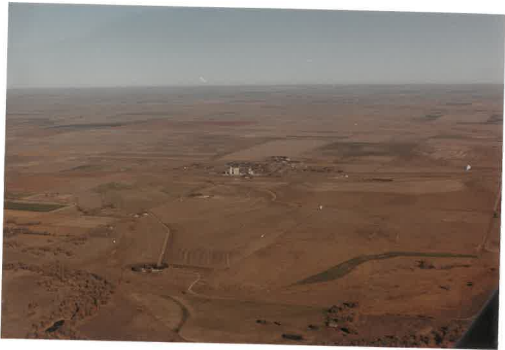
Photograph #1; looking north northwest.
