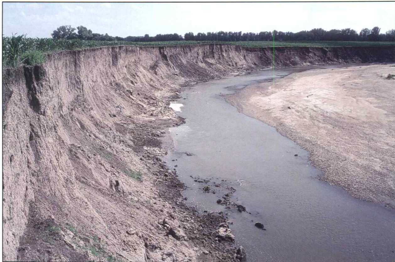
FIGURE 2-14. View of the cutbank at the Old Bridge site.
