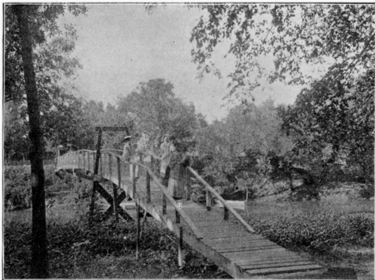
Suspension Bridge, Louisville.
