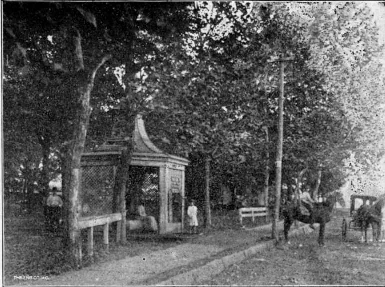
West Pavilion, Baxter Springs.
