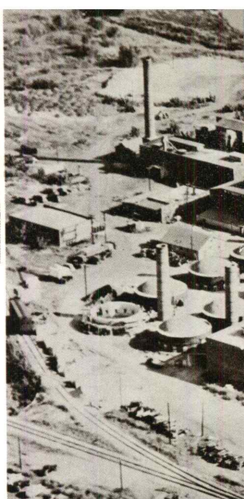
Pittsburg, Kansas, plant of W. S. Dickey Clay of clay pipe. Nearby pit where raw clay is obtained. Clay is one of our low-unit-value commodities, clay is the basis of many products (see page 26) and has high potential for extended production possible by modern scientific equipment (example below).
