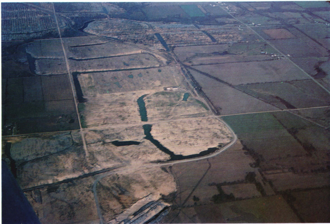
Plate 1. An aerial view from the south showing the mine site, December 1975.
