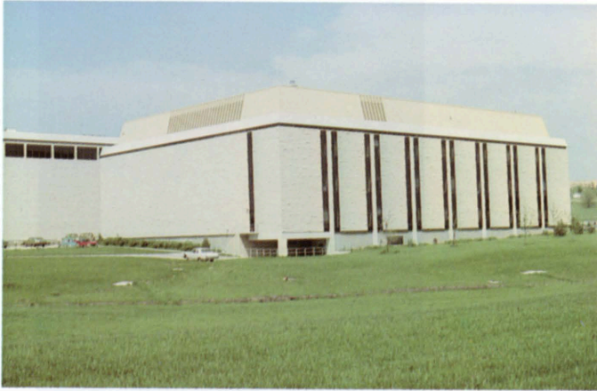
Fig. 43 - Cottonwood cut stone and Silverdale split-face stone were used to form part of the veterinary medicine building at Kansas State University in Manhattan.
