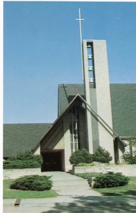
Fig. 25 - The Cresswell member of the Winfield Limestone was used to build Trinity Lutheran Church at Winfield.
