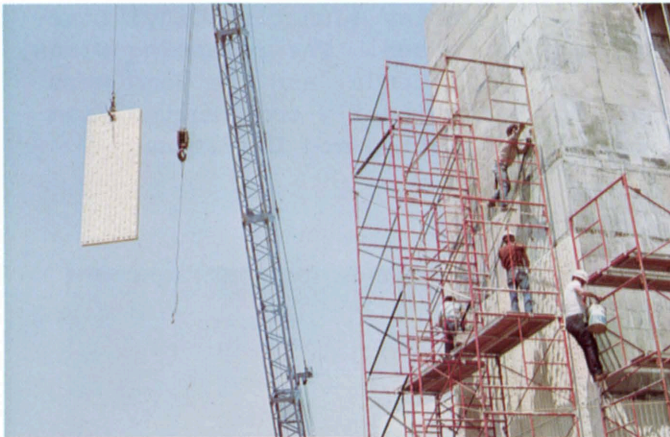
Figs. 12 and 13 - Two photographs showing the positioning of a fluted Neva Limestone panel on the new Engineering building at Kansas State University.
