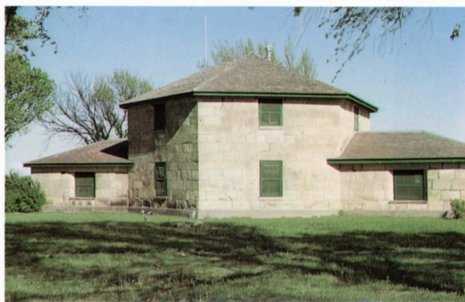
Figs. 16 and 17 - Fort Hays Limestone was used to construct the blockhouse at Fort Hays (Hays, Kansas). The second photograph clearly shows the saw marks on the individual blocks.
