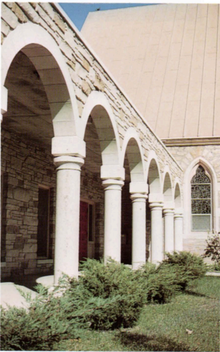
Fig. 30 - Cottonwood Limestone columns along a portion of the Trinity Episcopal Church at Lawrence.
