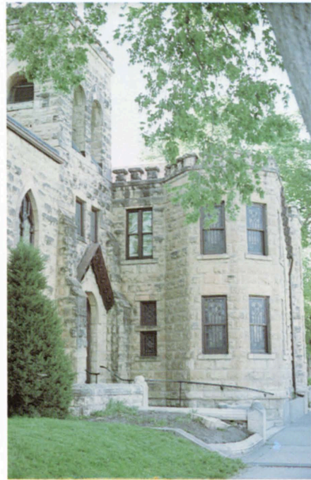
Fig. 19 - A portion of the First Southern Baptist Church at Abilene constructed in 1876 from Cottonwood Limestone.
