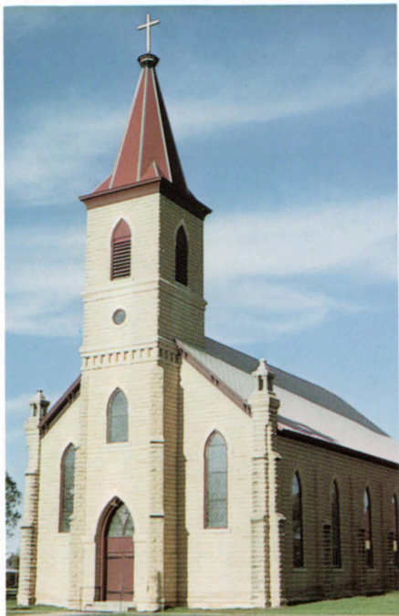
Fig. 20 - Saint Joseph's Church at Liebenthal (south of Hays) was built in 1902 from Fencepost Limestone
