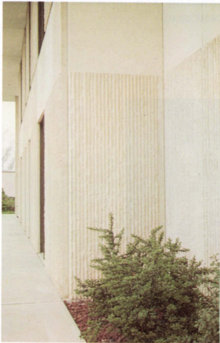
Fig. 52 - Fluted Onaga limestone panels add an interesting texture to the Hackler Office building in Olathe.
