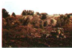
Leveling with bulldozer.
