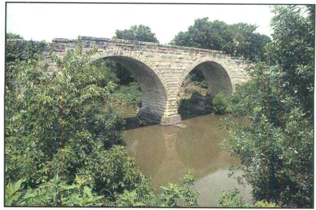
Bridge built of Cottonwood limestone near Elmdale, Chase County.
