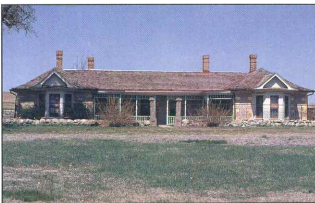
Cottonwood Ranch near Studley (Sheridan County), built of rock from the Ogallala Formation and Niobrara Chalk.
