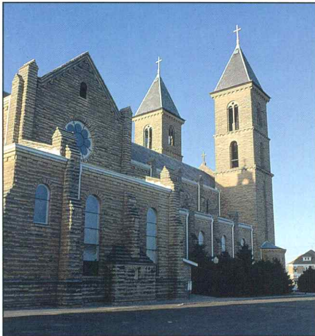
St. Fidelis Church (Cathedral of the Plains), Victoria, is built of Greenhorn Limestone, a common building stone in north-central Kansas.
