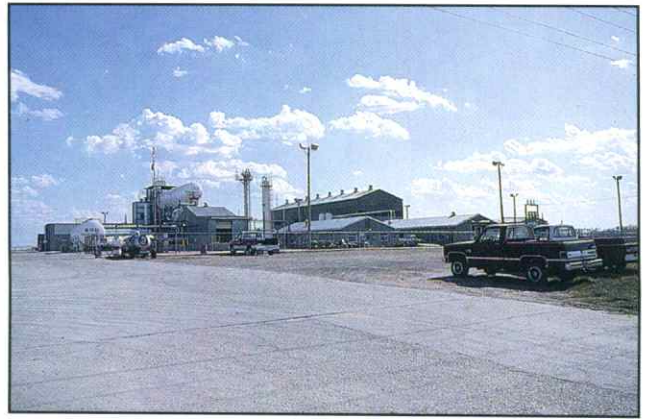
Helium plant at Otis, Rush County.
