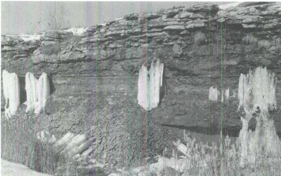
Ground water, moving along an underground layer of rock, leaves the subsurface and freezes at this Johnson County roadcut.
