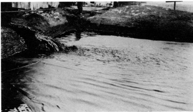
FIGURE 33 (right)—THREE VIEWS OF THE CONSTRUCTION OF A 55,000-BBL OIL-STORAGE TANK ON the Roubach lease in 1935. The tank was reported as filled in 12 days with oil flowing from the Roubach No. 1, or 4,583 BOPD; photographs courtesy KIOGA.
