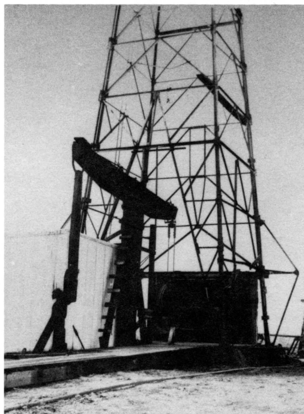
FIGURE 34a (below)—PHOTOGRAPH OF THE ROUBACH LEASE, 1935, FROM THE TOP OF THE 55,000-BBL STORAGE TANK. Shows the Roubach No. 1 derrick and the flat agricultural plains area. 34b (right)—CLOSE-UP OF ROUBACH NO. 1 PUMPING OIL. Note the steel (not wood) derrick and former cable-tool equipment left on location for production use in pumping oil; courtesy KIOGA.
