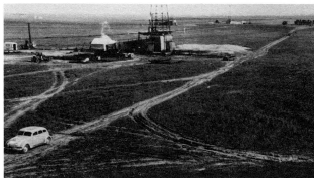
FIGURE 34a (below)—PHOTOGRAPH OF THE ROUBACH LEASE, 1935, FROM THE TOP OF THE 55,000-BBL STORAGE TANK. Shows the Roubach No. 1 derrick and the flat agricultural plains area. 34b (right)—CLOSE-UP OF ROUBACH NO. 1 PUMPING OIL. Note the steel (not wood) derrick and former cable-tool equipment left on location for production use in pumping oil; courtesy KIOGA.
