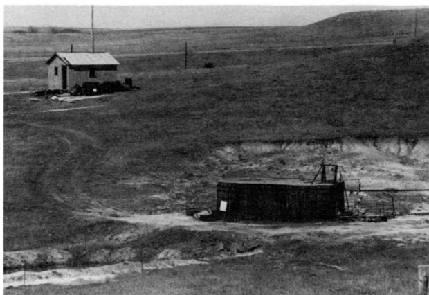
FIGURE 42—PHOTOGRAPH OF A DEEP SALTWATER-DISPOSAL (SWD) INSTALLATION. Disposal of brine into the Arbuckle formation, depth near 3,400 ft (102 m), is by gravity flow from the brine-storage tank. Courtesy Russell County Historical Society.
