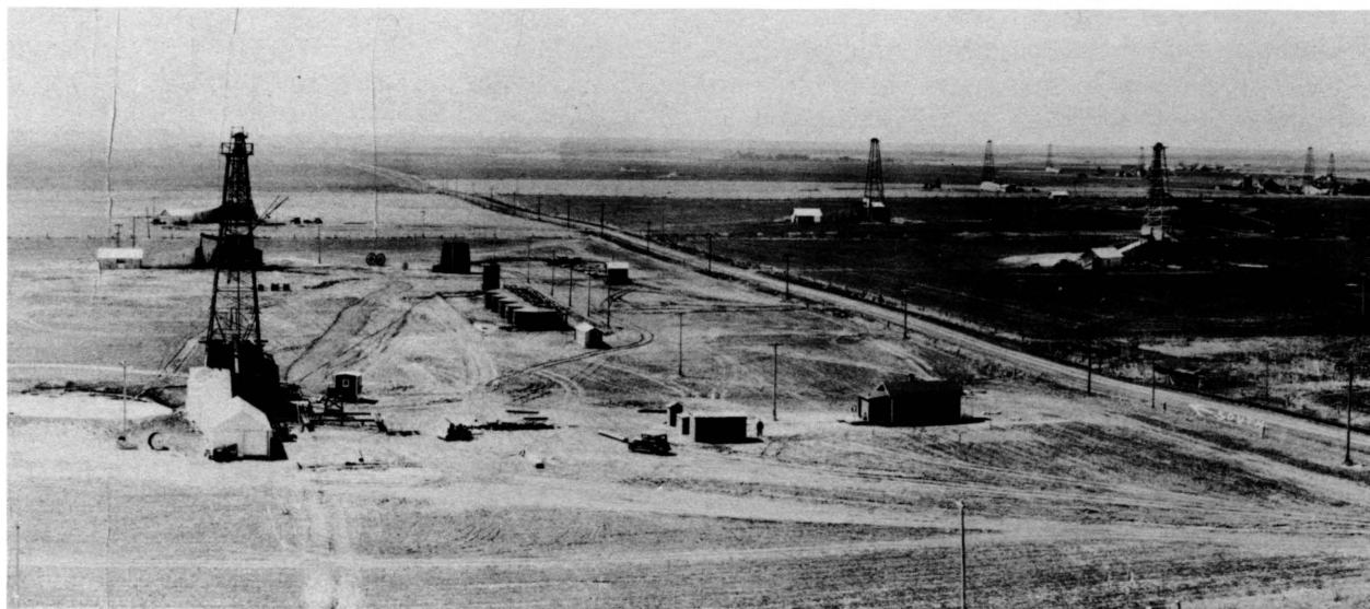
FIGURE 28—GORHAM OIL FIELD, APRIL 14, 1928, a portion of a panoramic photograph; view to the southwest. In the left foreground, Stearns and Streeter's Mermis No. 2 is testing the Gorham sand. Directly aligned behind it (south), the Mermis No. 1 is pumping 580 BOPD from the Gorham sand and south of it a third well, the No. 12 Mermis is drilling; courtesy Russell County Historical Society. See back cover.
