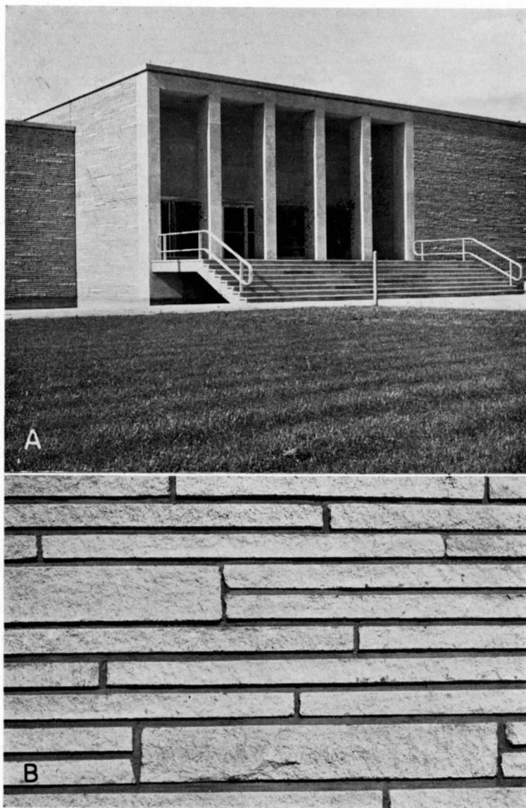
PLATE 10.—Funston Limestone ("Onaga" stone). A , Eisenhower Museum, Abilene, built of limestone in split-face ashlar pattern. B , Split-face ashlar finish on "Onaga" stone, Eisenhower Museum.
