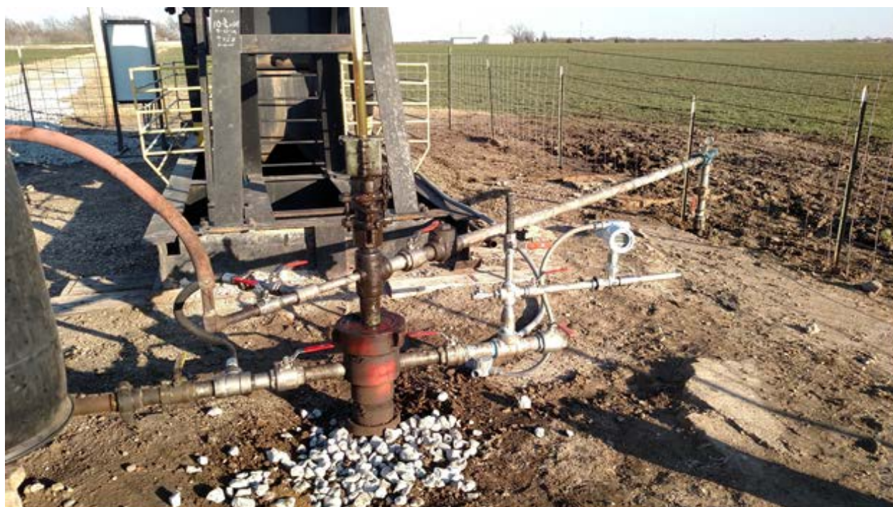
Figure 18. Flowmeter is now installed on #61 and #62 and soon on wells #53 and #69.
