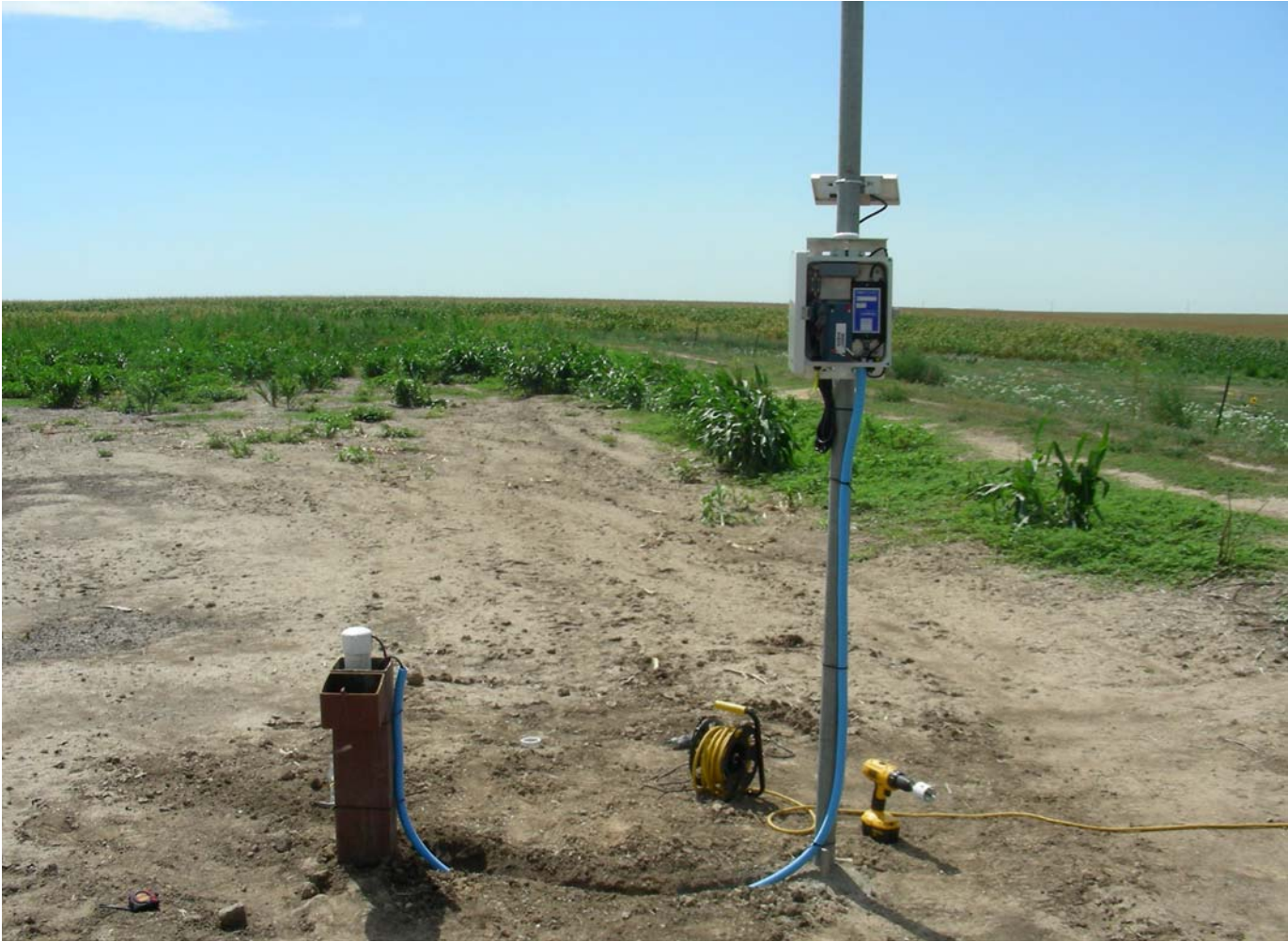
Figure 2. Haskell County site during telemetry installation.
