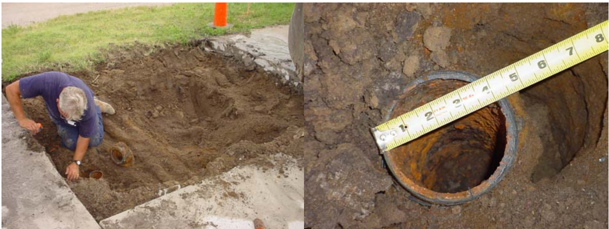
Figure 21. The total field component of the magnetic anomaly in grid U4 at the Union Salt site (top). The anomaly at (36, 40) is due to a probable utility pipe (4-inch) at a depth of 1 ft under 6 inches of concrete (bottom). Mike Cunningham of the City of Hutchinson is checking the pipe.
