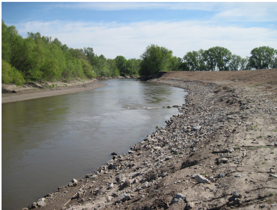
Figure 3—Neosho River stream bank after reshaping for stability. Photo: Kansas Water Office and The Watershed Institute.
