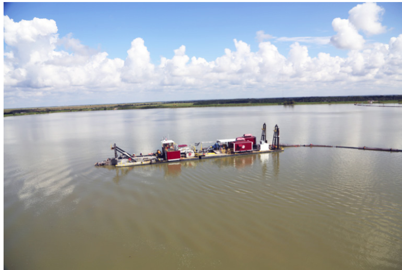
Figure 4—Hydraulic dredging with slurry pipeline. Photo: Great Lakes Dredge and Dock Company.
