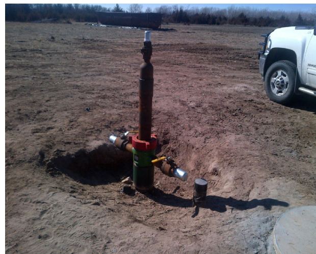
Figure 3—Retrofit drilling, injection wellhead and emplacement process of UCS's Class V well (Pangburn, 2013).
