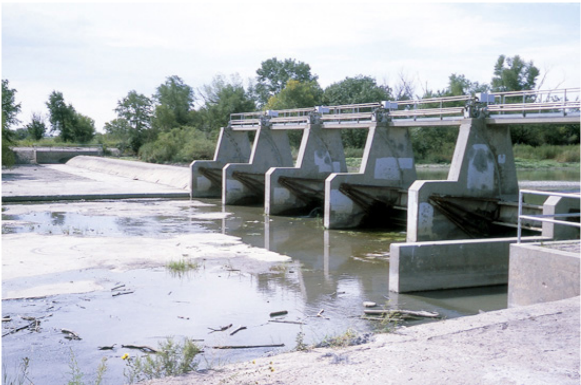
Figure 1—Dam on the Arkansas River near Dundee southwest of Great Bend used to divert water to Cheyenne Bottoms Wildlife Area.
