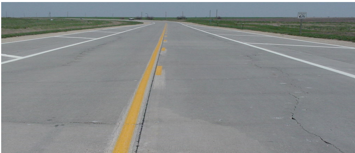
Figure 4-12. US-56 concrete pavement cracks after ettringite formation.
