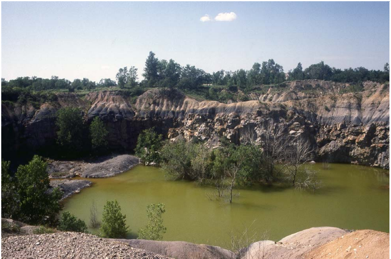
Figure 3-8. One of two large subsidence pits at the Sunflower mine (photo by Jim McCauley).
