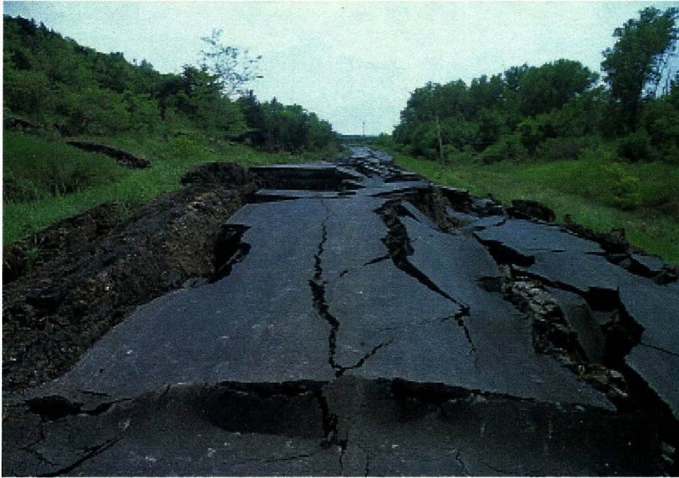
Fig. 4-5—Kansas landslides have damaged or destroyed houses and other structures, closed roads, and disrupted transportation systems. In May 1995, a landslide just south of Manhattan closed McDowell Creek Road and subsequently cost Riley County $880,000 to stabilize the slope and repair the road. The landslide, which occurred following several weeks of heavy spring rains, damaged over one-quarter mile of the road. The road was displaced about 20 feet vertically and 40 feet horizontally by the slide. The asphalt was pushed together in some places and pulled apart and twisted in others. Power poles moved laterally and were sitting at angles, the lines stretched taut. Many trees slid sideways but remained upright.
