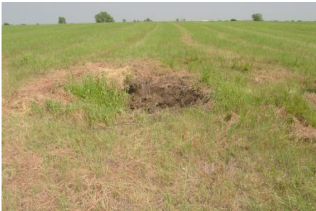
Image 1.—Backfilled sinkhole SW 34-25-06E, north view direction, by S Koontz, BCCD, July 2008
