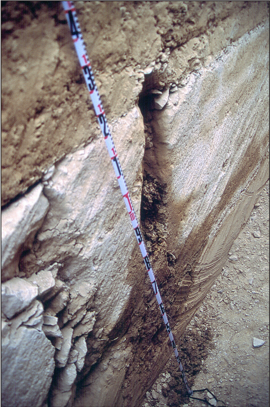
Figure 5. Close-up of a vertical joint. This joint was dripping water about four hours after the trench was excavated.
