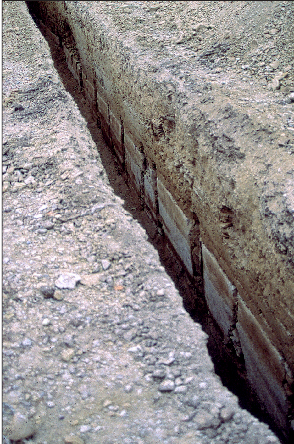
Figure 4. View of the east side of trench. Note the regularly spaced vertical joints in the limestone.
