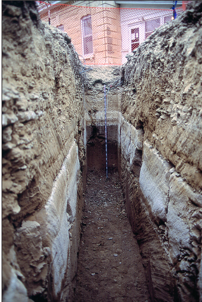
Figure 3. Limestone layer (2.4 feet thick) in waterline trench southwest of Ranch House. This is the upper limestone in Cross Section A-A'.
