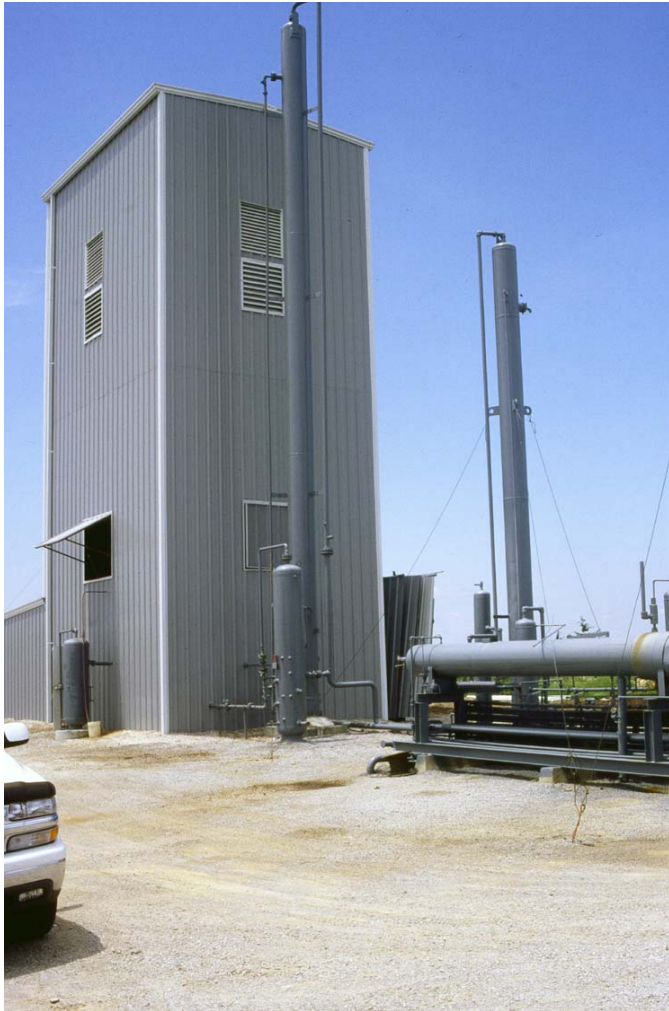
Figure 3. Dehydrator tower used by Dart Cherokee Basin Operating Co. to remove moisture, and minor impurities from the coal gas prior to passing through the Tallman Compressor Station. The tower is adjacent to the Tallman compressor.
