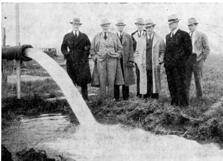
FIGURE 5. View of discharge from the first Wichita city well in the new supply area near Halstead. The well is discharging 1,600 gallons a minute through a 10-inch orifice, and the draw-down at the close of a 36-hour pumping test was 28 feet.
