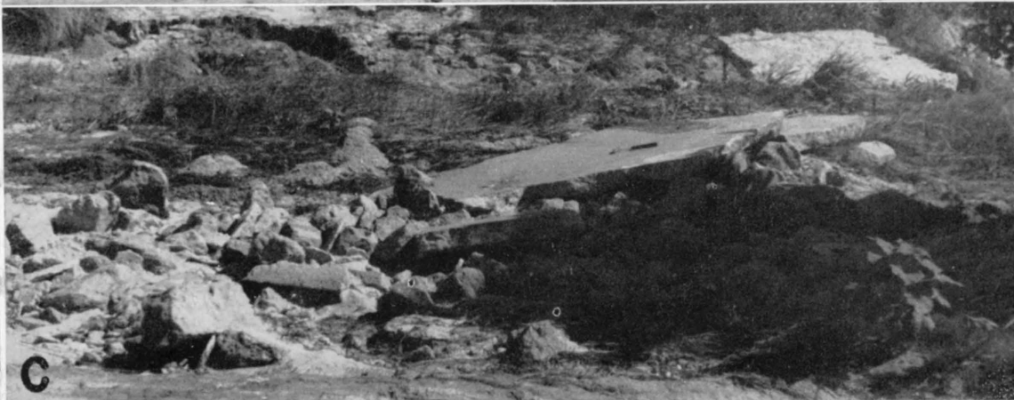
PLATE 31. A. Imbricate blocks in channel of Bluff creek. B. Imbricate blocks in the bank along Bluff creek. C. Concrete slabs carried downstream by abnormal overflow waters after the breakup of the spillway of the dam at Meade County State Lake. The water moved from left to right. This illustrates the way in which the imbricate blocks were probably deposited. (pp. 171-172.)
