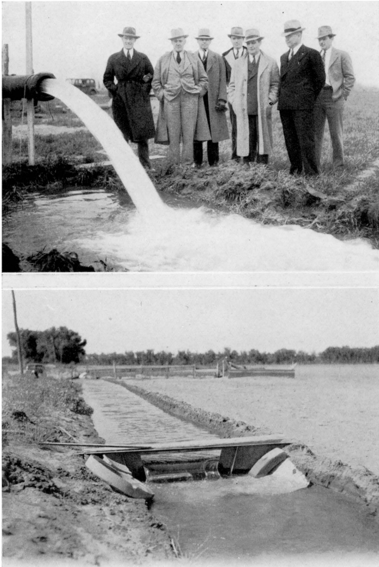
PLATE 11. Upper , The first Wichita city well in the new supply area near Halstead, located by Geological Survey investigations. This well tested 1,600 gallons a minute; the flow is from a 10-inch orifice. The drawdown in the well at the close of a 36-hour pumping test was 25 feet. Lower , Measuring the flow of water obtained from shallow wells in the Arkansas river alluvium near Dodge City (Geological Survey in cooperation with Division of Water Resources). (S. W. Lohman, H. A. Waite.)
