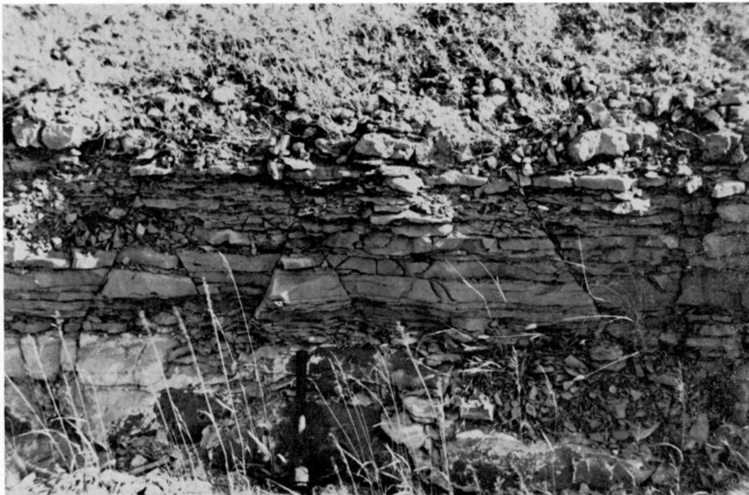
FIGURE 4.—Joint traces of Sets I and II dipping between 65° and 70°; Herington Limestone; E½ NE¼ NE¼ sec. 30, T. 24 S., R. 4 E.
