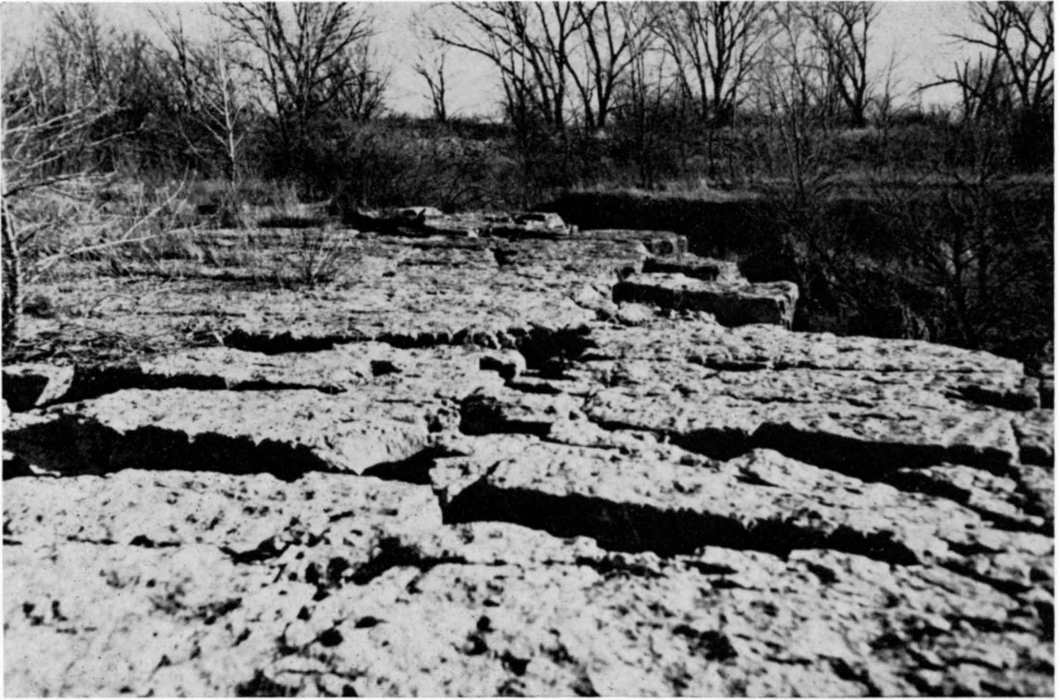
FIGURE 11.—Open joint traces resulting from advanced solution of limestone; Set II joint extends into picture while Set I joints are perpendicular to it; Winfield Limestone; NE¼ sec. 13, T. 27 S., R. 3 E.
