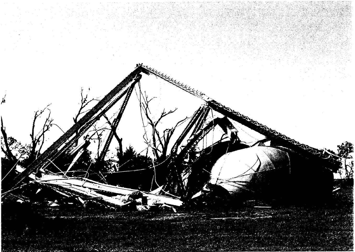
WATER TOWER AFTER TORNADO 5/31/08
