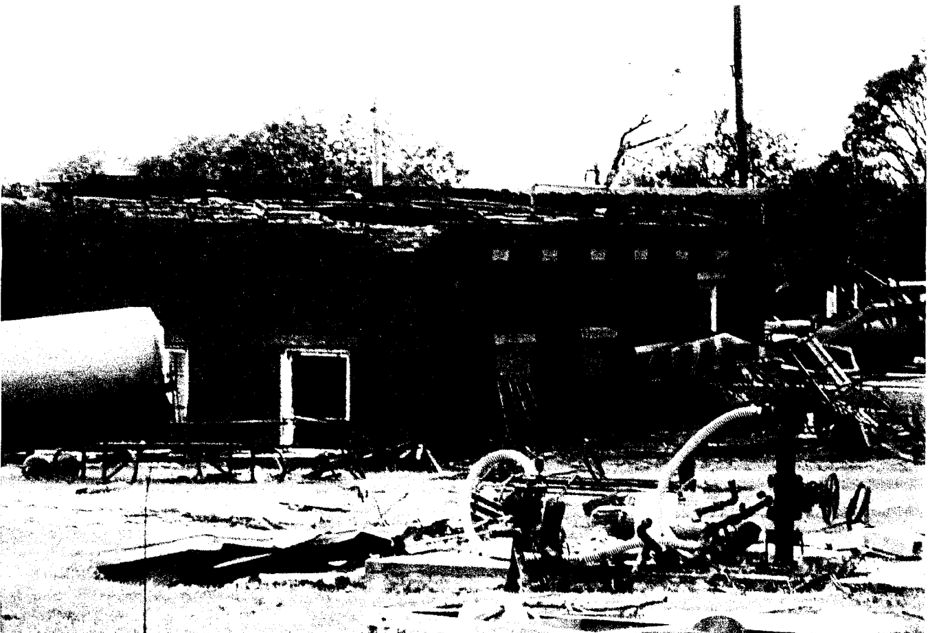
VIEW TO WEST OF CHLORINATION PUMP STATION & CITY SHOP
