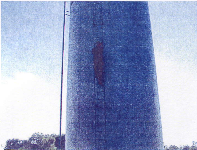
Climbing the tower, mid-way up.
