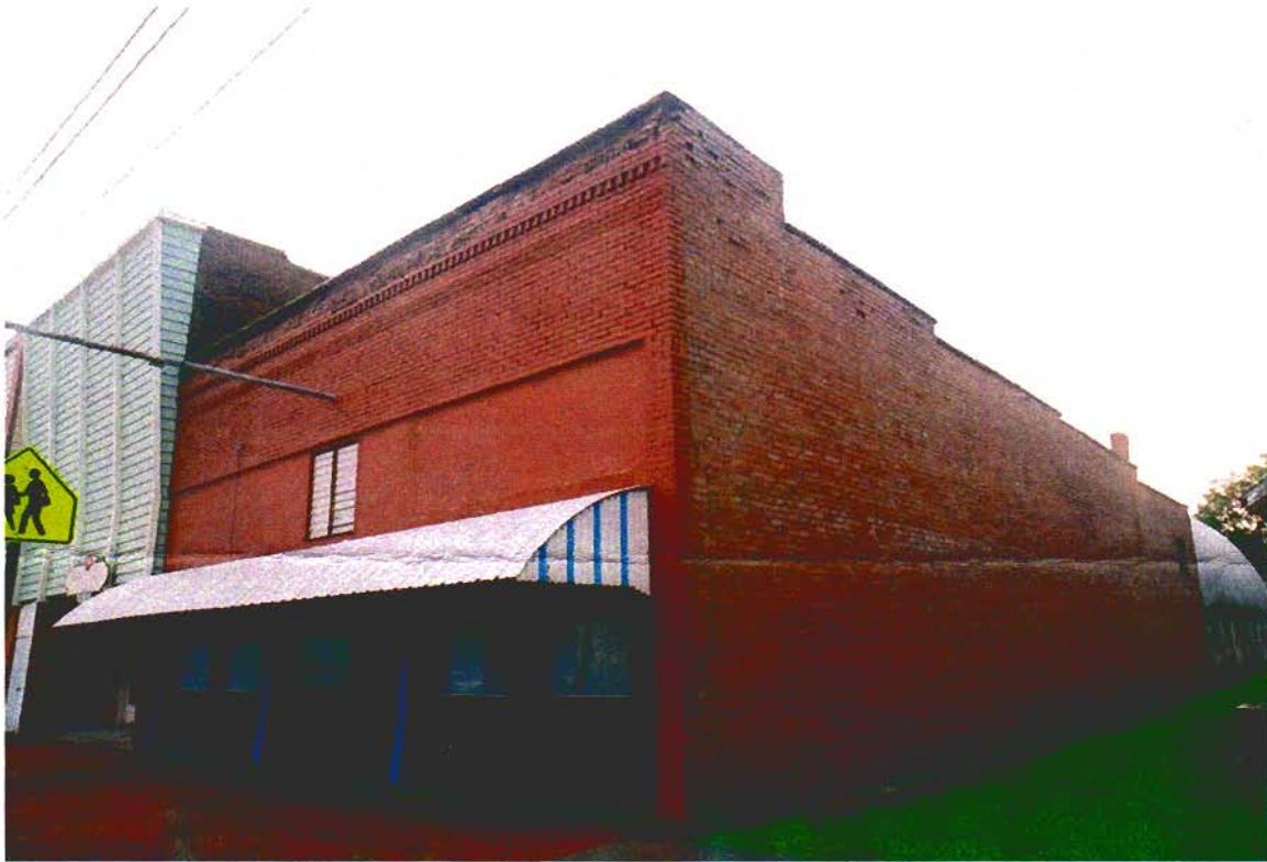
Exterior view of the building located at 111 South Main Street, Erie, Kansas.
