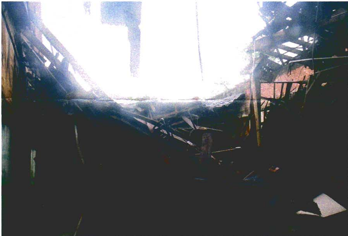
Interior view of the building located at 111 South Main Street, Erie, Kansas.
