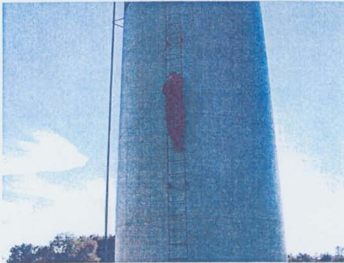
Climbing the tower, mid-way up.
