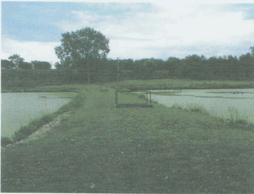
CENTER DIKE, LOOKING SOUTH RAILROAD IN BACKGROUND
