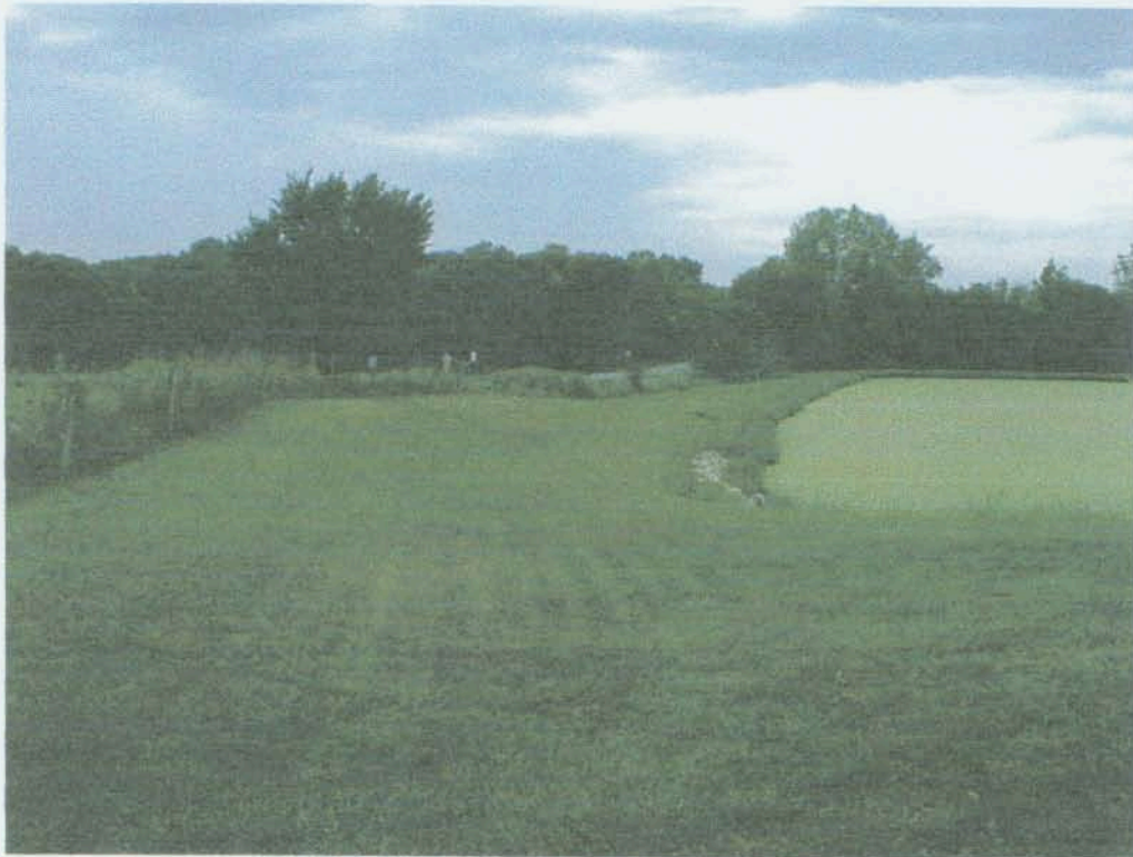
WEST SIDE OF EXISTING CELL NO. 1 COUNTY ROAD TO THE WEST
