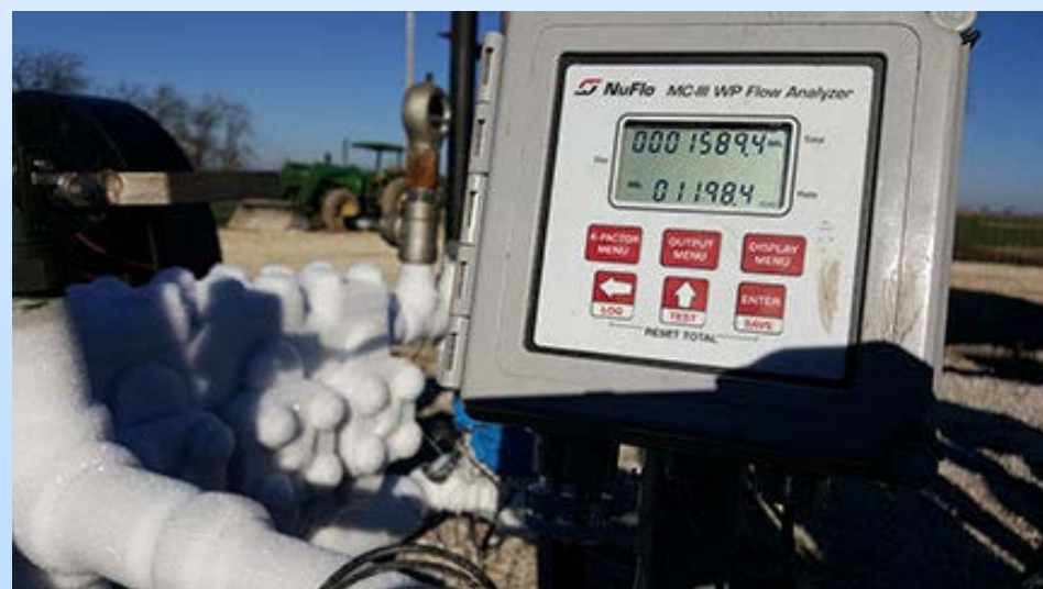
SCADA System installed on wells
