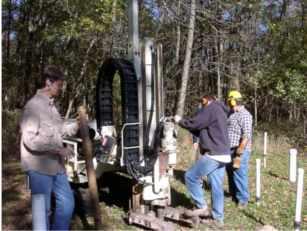
Figure 20. Direct push installation of the new wells.
