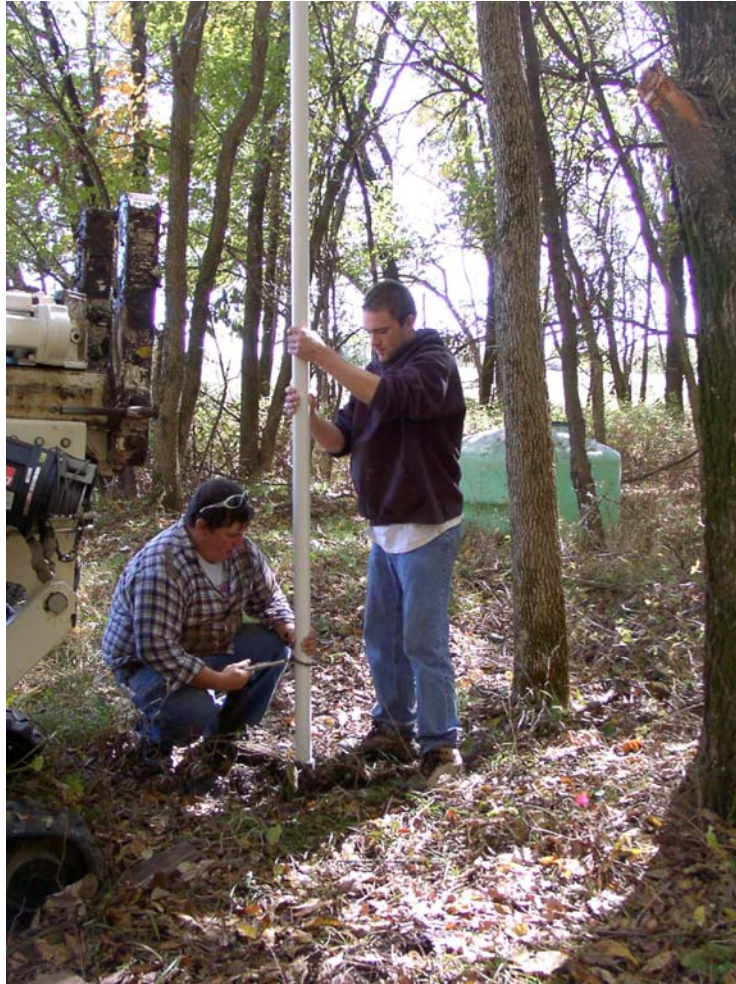
Figure 22. Installation of casing in new wells.
