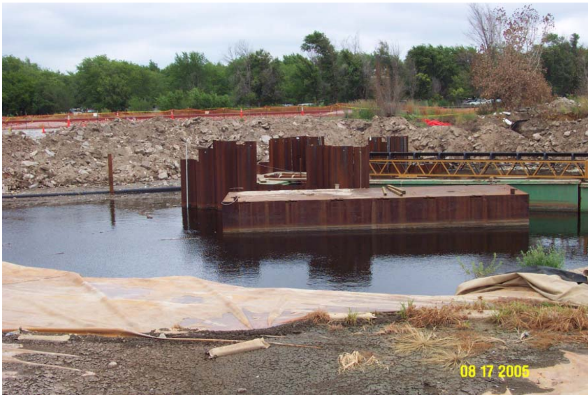
Installed framing used by consulting firm for filling sinkhole. Looking north towards Burlington Northern-Santa Fe railroad tracks. S. Ausbrook, August 2005.
