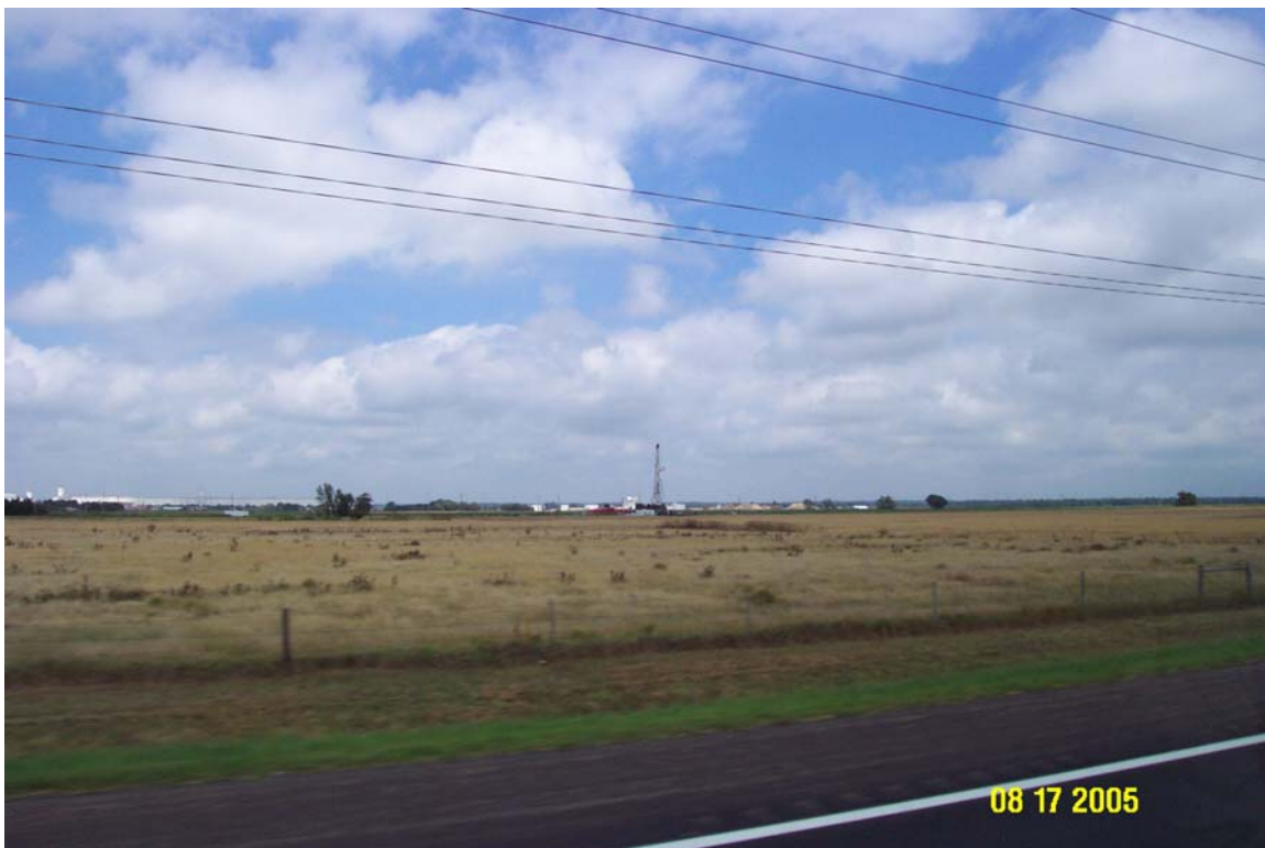
East of Hutchinson, KS Highway 50. Well drilling for new disposal well for salt water. S. Ausbrook, August 2005.
