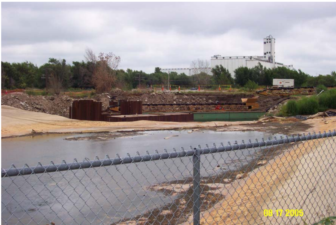
Hutchinson old Carey salt plant sinkhole. Looking north towards Burlington Northern-Santa Fe railroad tracks. S. Ausbrook, August 2005.
