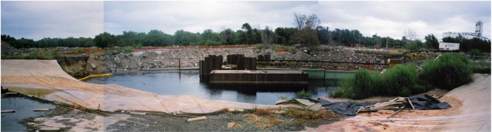
Cross-section of sinkhole at old Carey Salt plant, Hutchinson, KS. M. Townsend, August 2005.
