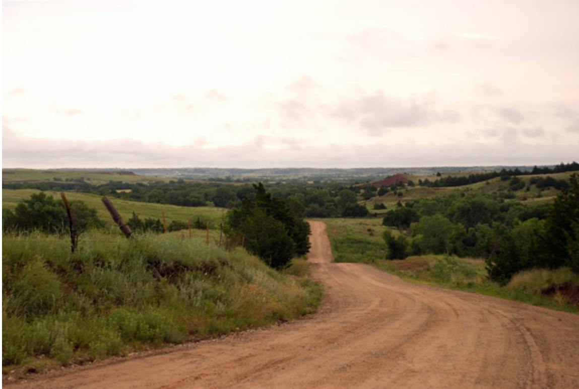
Figure 2—Many roads in the area of the Mississippian limestone play are unpaved and not built to withstand heavy truck traffic.
