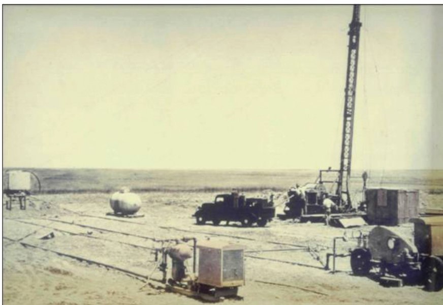
Figure 1—First experimental fracturing job conducted in 1947 by Stanolind Oil in the Hugoton gas field of southwestern Kansas utilizing “1,000 gallons of naphthenic-acid and palm-oil- (napalm-) thickened gasoline” . . . “and sand from the Arkansas River” (from Montgomery and Smith, 2010, p. 2).
