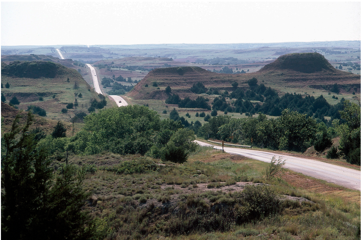
Figure 1—U.S. Highway 160 running through the Red Hills in Barber County.
