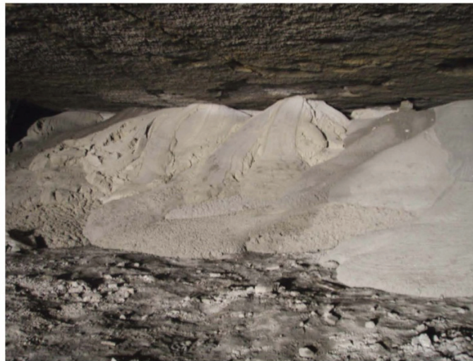
Figure 3. Containment wall for grout backfill (photo courtesy HNTB).
