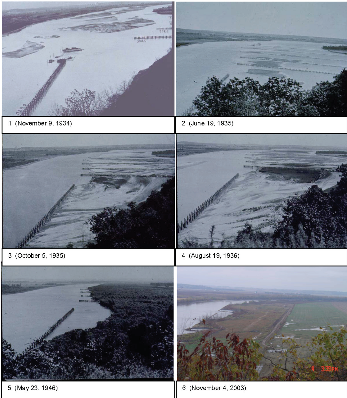
Figure 5. Time series of photos over a period of 69 years showing construction and filling of a dike field (Cardno Entrix, Inc., 2011).
