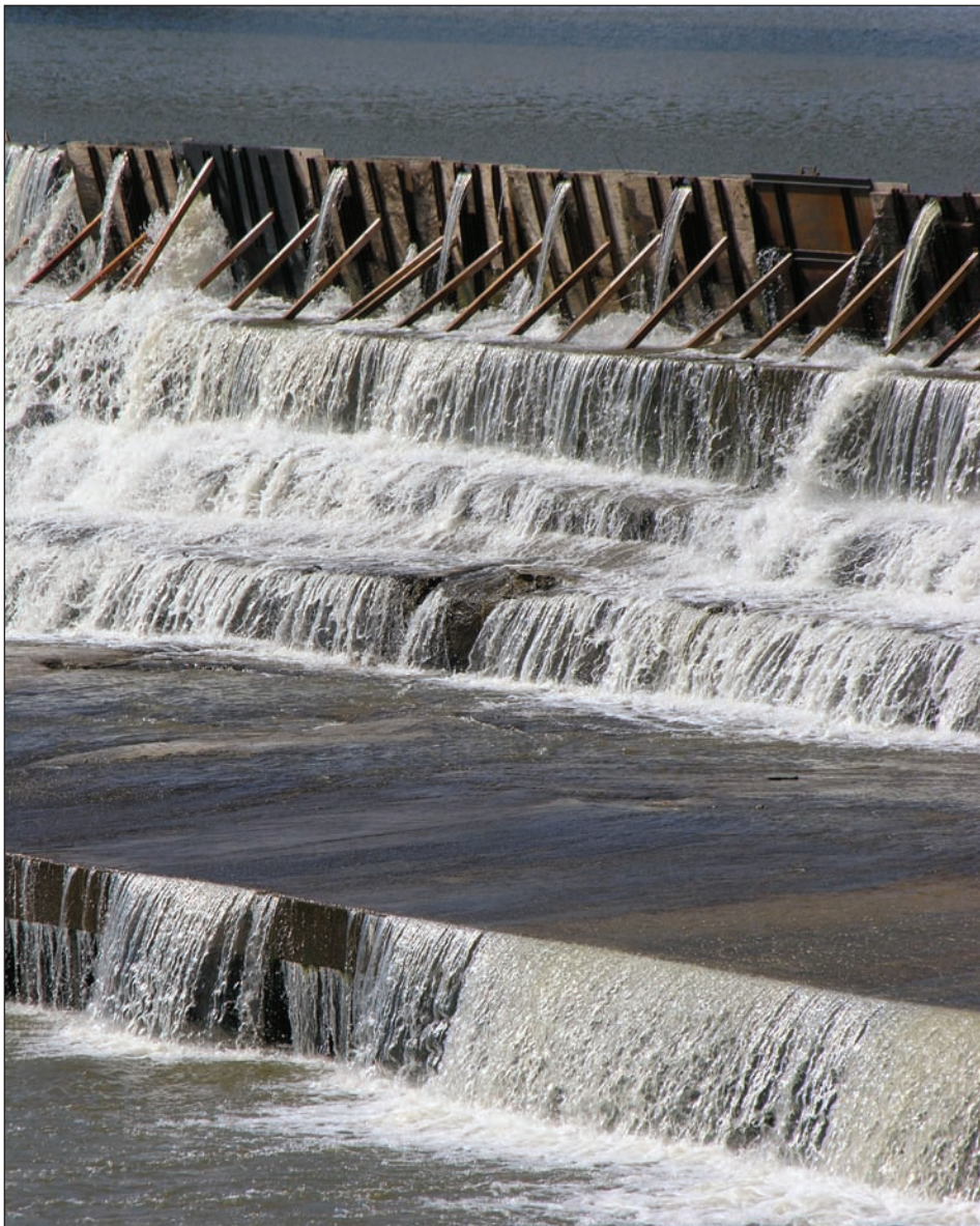
Figure 2. Flashboards on Bowersock dam (photo by Cathy Evans).
