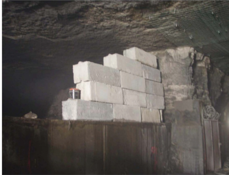
Figure 3. Containment wall for grout backfill (photo courtesy HNTB).
