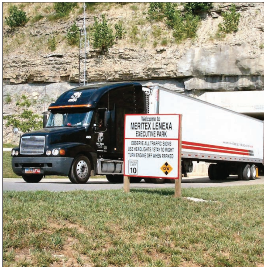
Figure 1. Portal entrance to the Meritex facility in Lenexa, Kansas, within the Argentine Limestone Member (photo courtesy Meritex).
