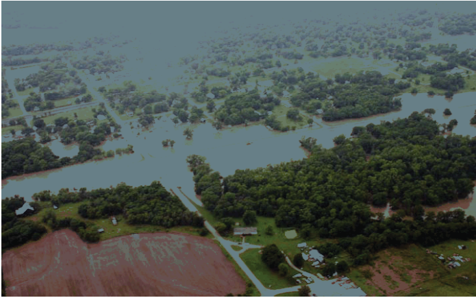
Figure 2. 2007 flood, looking west toward Altoona (photo courtesy of the KWO).
