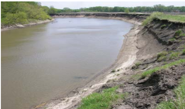
Figure 2. Cut bank and sediment erosion on the Neosho River upstream of John Redmond Reservoir near Neosho Rapids. (Photo by Bob Sawin, Kansas Geological Survey).
