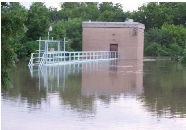
Figure 1. Independence water-treatment plant during 2007 flood (photo courtesy of the KWO).
