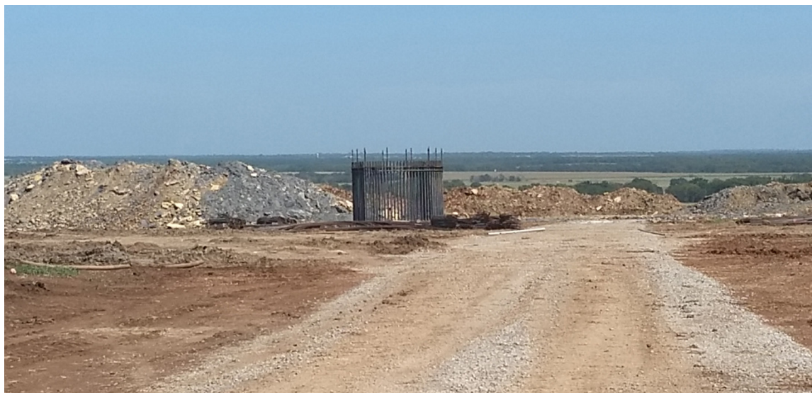
Figure 5. Steel lattice foundation of a new wind turbine at Jayhawk Wind Energy Center.
