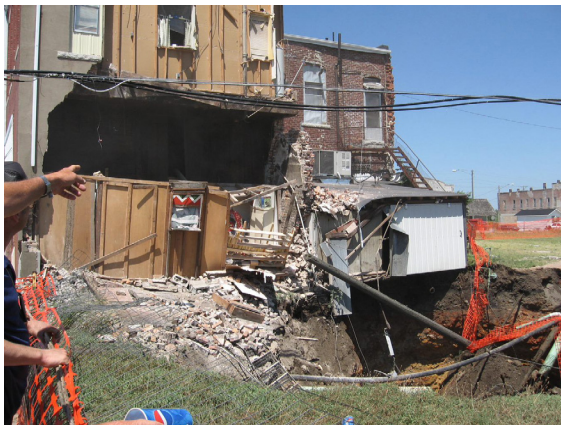
Figure 13. Sinkhole that opened in Galena in 2009. Damage to apartment building (top), and interior view of sinkhole (bottom). (Source: Kansas Department of Health and Environment Superfund Program.)
