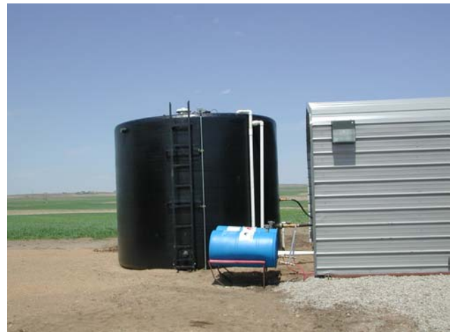
Figure 6. CO2 pilot water injection tanks with treatment chemicals.
